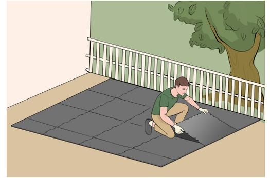
Start laying out the panels according to the layout diagram. “Staging” the panels allows them to acclimate to the ambient temperature as well as the adjacent panels. This also allows different crews to stay busy: one laying out panels and one snapping them together.
