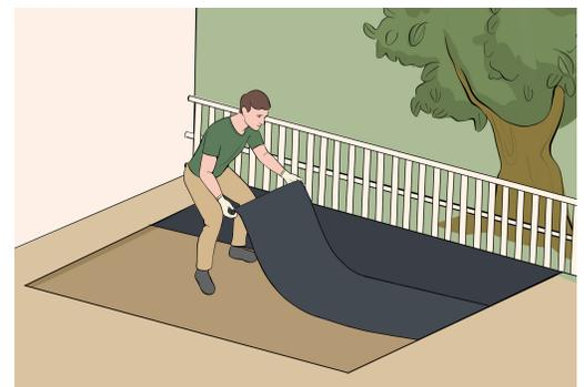
Take care to overlap a minimum of 6”. Pay attention to apparent water flow direction when overlapping the fabric.
